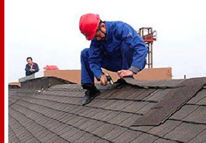
3. Fix the panel with tile nail
